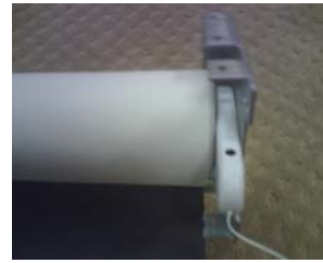
Motor installed to bracket
