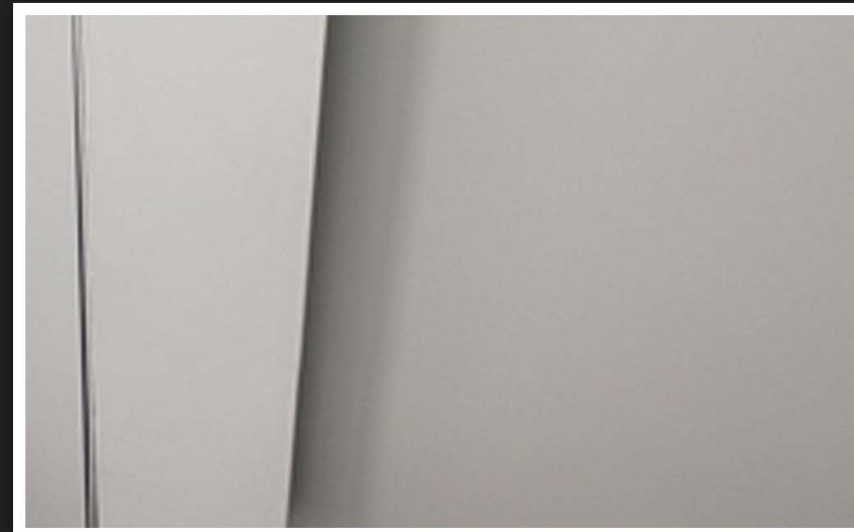
Uneven gaps from wavy drywall
